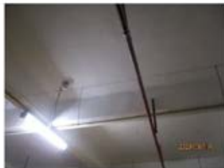
13. Fire sprinkler system and smoke detector
